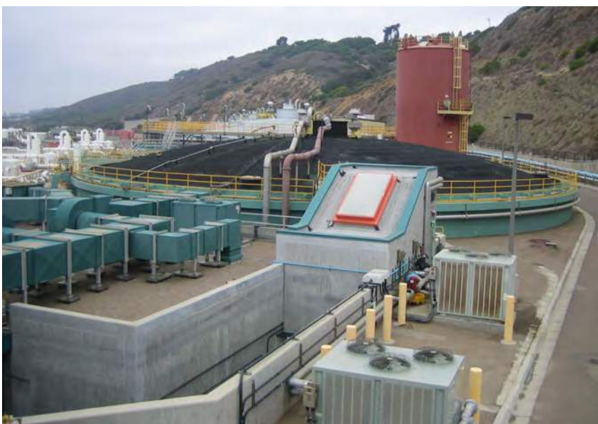
Collection of methane gas at Point Loma Wastewater Treatment Plant
