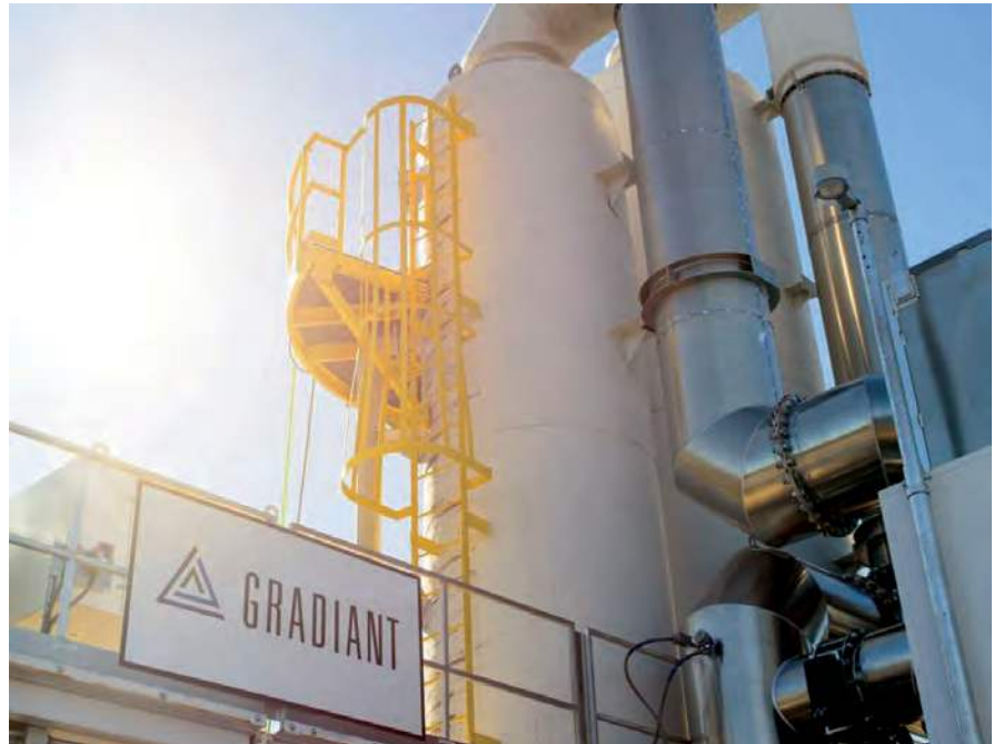
Gradiant industrial water treatment facility
