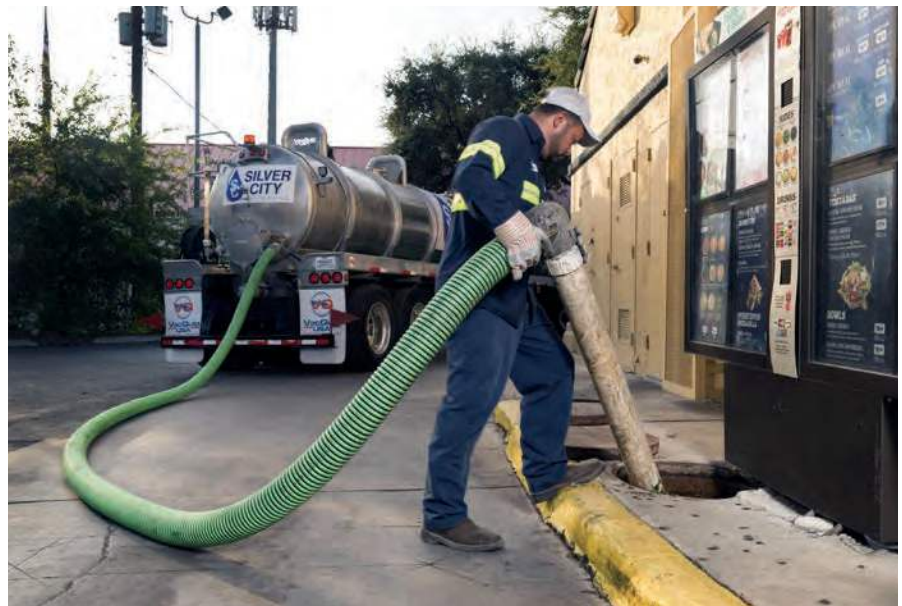
Waste Resource Management removes grease trap waste from the wastewater treatment system
