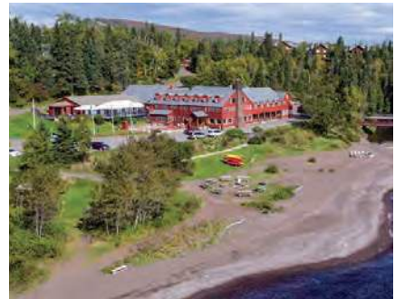
NSU wastewater treatment at Lutsen Resort in northern Minnesota
