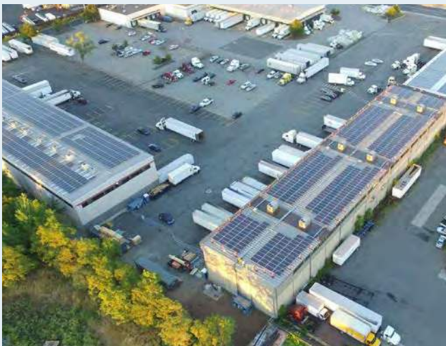
1.2 MW rooftop solar project in Suffolk County, Massachusetts
