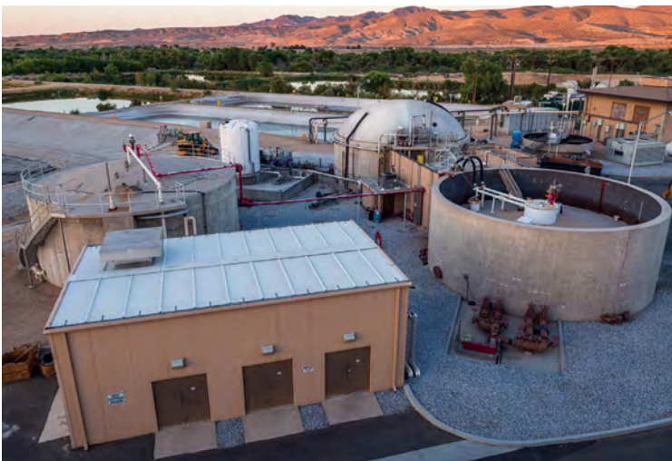
Victor Valley Wastewater
