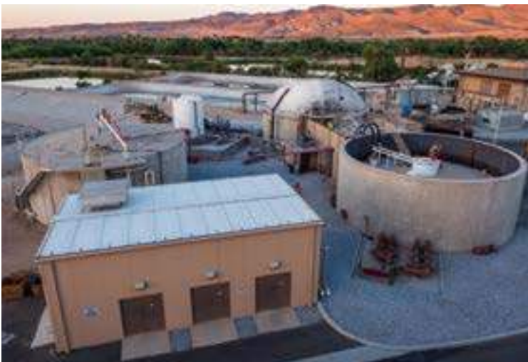
Victor Valley Wastewater
