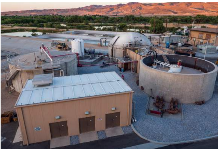
Victor Valley Wastewater
